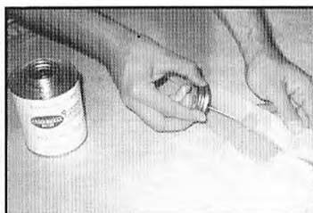
6 Weld all seams and corners using Composeal Solvent Cement for flexible PVC
