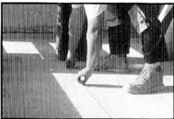
1 Carefully lay out installation to minimize cuts and seams. Chalkline sheet locations
