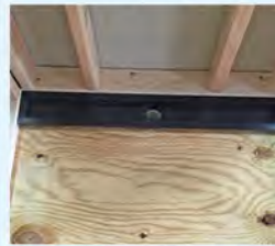
Side & back flange flush to rough framing
