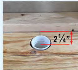
Correct placement of drainpipe
