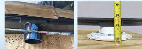
Can cut drain outlet to minimize elevation
